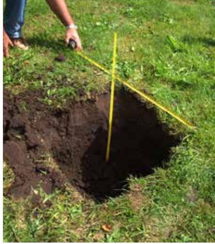
Dimensions of holes: e.g. 50 x 50 x 75 cm (see the following pages).
