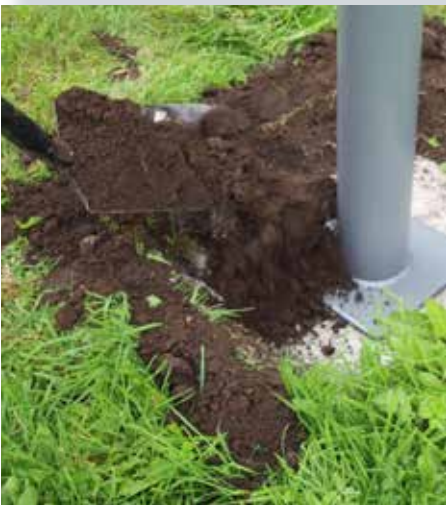
Make sure the fitness station is stable and properly fastened before filling with dirt to the surface.
