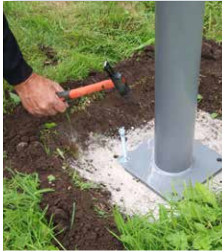
Mount the M12/M16 concrete bolts.
