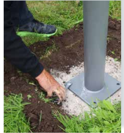
Tighten the anchors (M12 = 90 N/m and M16 = 120 N/m).
