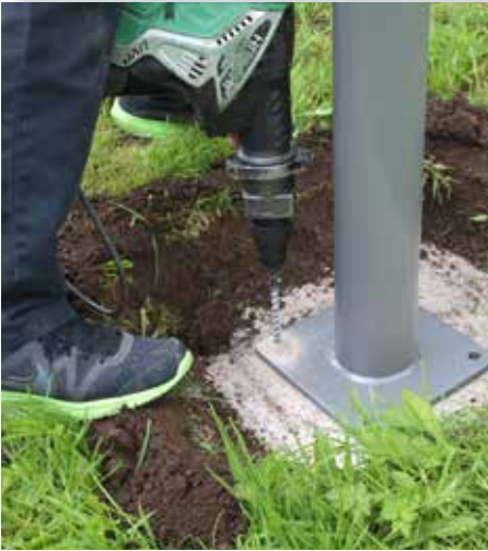
Drill bolt holes with a concrete hammer.
