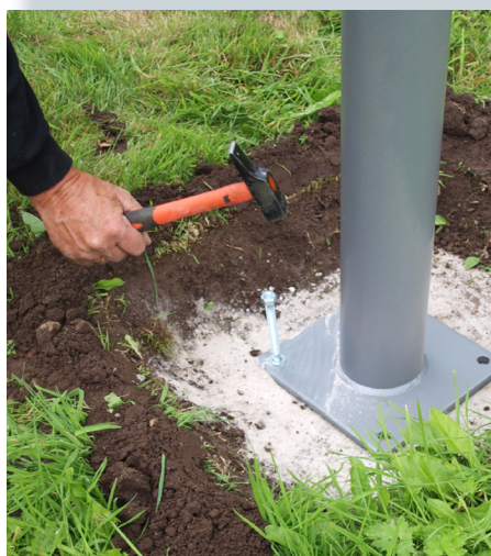
Mount the M12/M16 concrete bolts.
